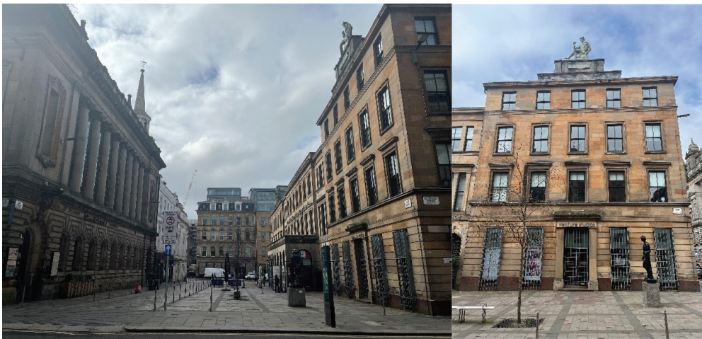
Figure 4. Refurbished façade with the sculptures on the roof.
