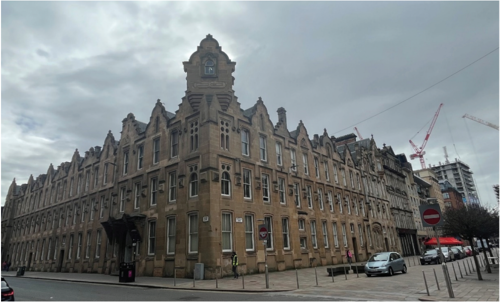
Figure 1. The façade was designed by Robert William Billings. 26
