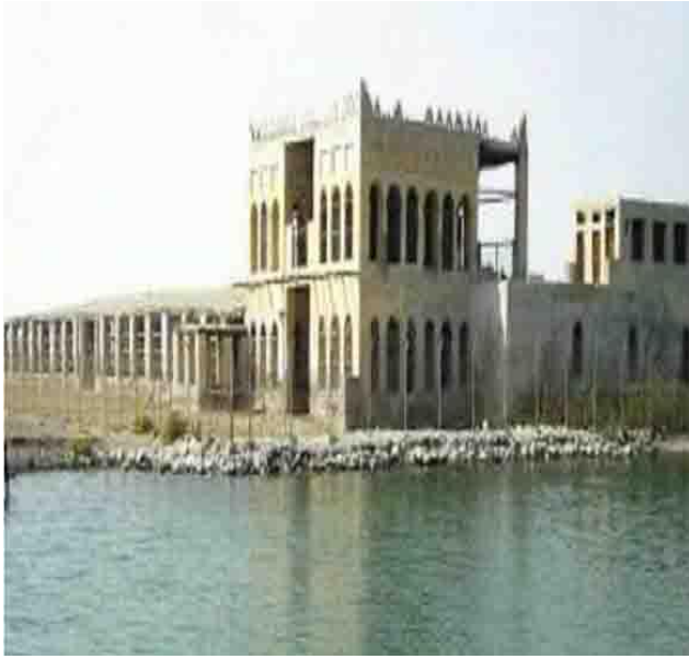
Figure 2.8: An image of a traditional home in the Eastern Region on the costal side. Source: King, 1998.
