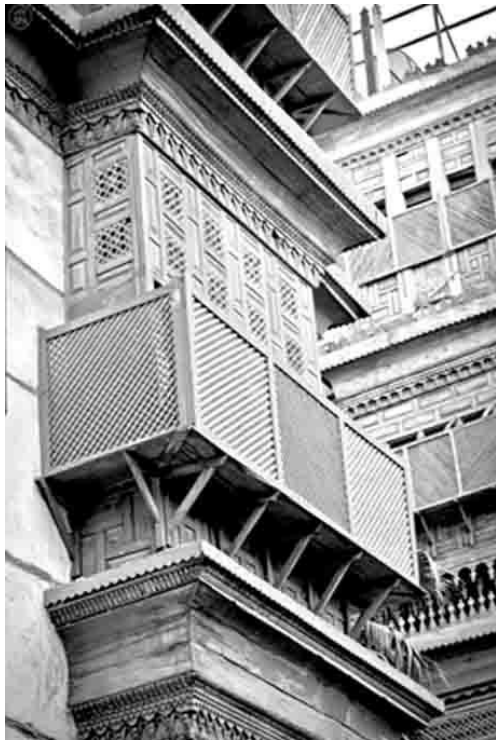
Figure 2.6: An image of wood screening ( rowshan ). Source: Ragette, 2003.
